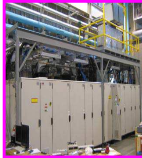
5 MW Converter "Amplifier"
