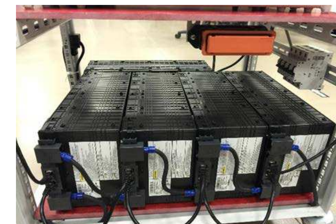
5 Toshiba LTO batteries connected in series with protection circuitry
