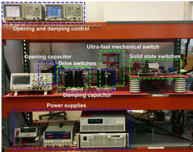
Fig. 14. Test setup of the active damping method.
