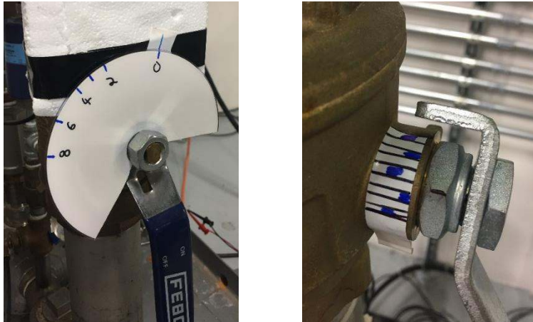
Figure 4. Ah hoc measuring tools for suction (left) and discharge (right) valves
