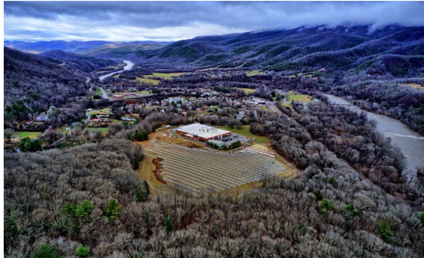
Duke Energy Hot Springs Microgrid Hot Springs, Madison County, North Carolina
